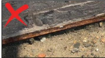
Example of a rusted drip edge that has failed.
