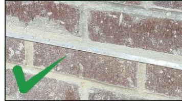
Example of a Type 304 stainless steel drip edge.
