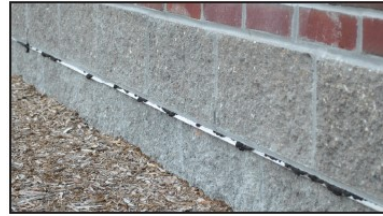
Examples of rubberized asphalt that have reached the flow temperature.
