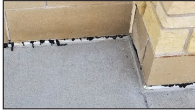
Examples of rubberized asphalt that have reached the flow temperature.
